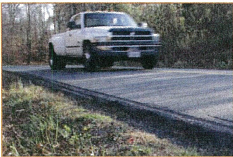
Edge drop-off on a rural road.
